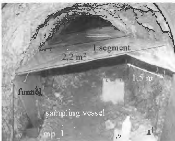
Fig. 3 Construction for collecting water samples.
