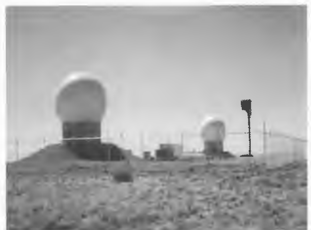
Fig. 5 Gateway Earth Station (GES). Source: http://www.orbcomm.com .
