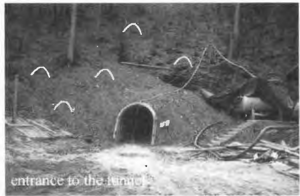
Fig. 9 View on the entrance of the tunnel.
