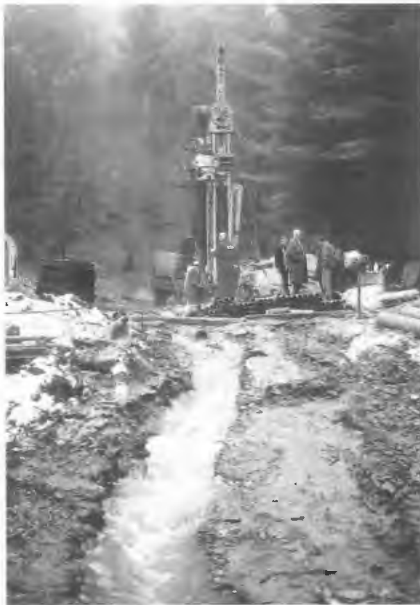
Sl. 3 Karotaža bušotine Lo-5. Fig. 3 Logging of the borehole Lo-5.
